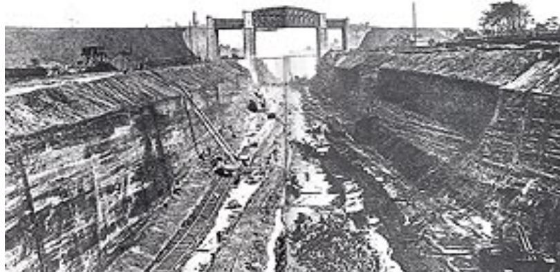
The Canal under construction near Latchford, Warrington, 1890
