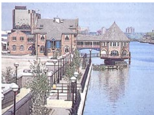
Trafford Wharfe today: Wharfeside Promenade.
