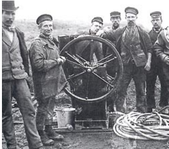
Diving team with pump at Thelwall, November 1890
