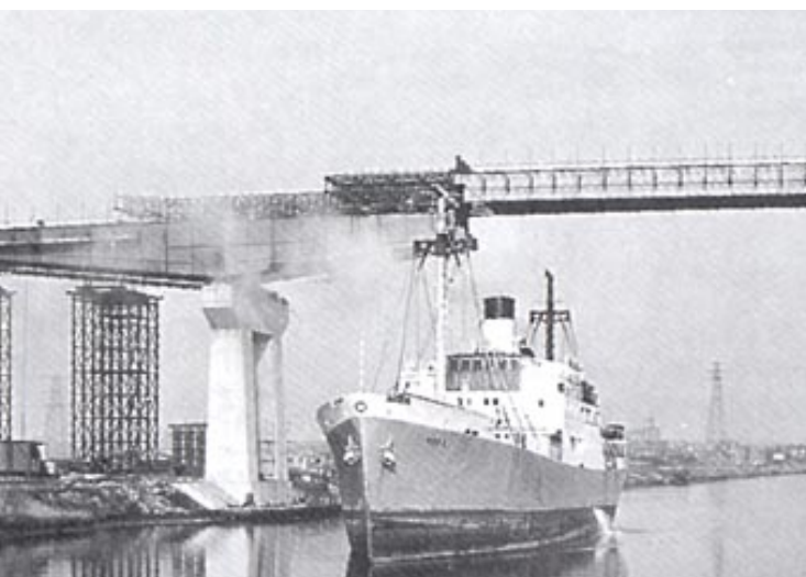
Barton Bridge for Lancashire Circa 1960
