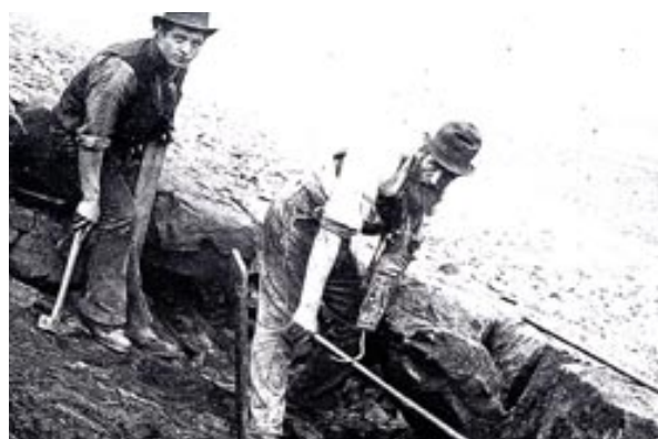
One-armed navy at work. It was inevitable that during the construction of the Canal, some workers would suffer serious accidents. A chain of first aid stations and three base hospitals (temporary buildings of timber) were strategically sited along the line of the Canal, and a Liverpool orthopaedic surgeon, Robert Jones, later to become Sir Robert Jones, was appointed to supervise what is thought to be the first organised accident service in the history of British surgery.
