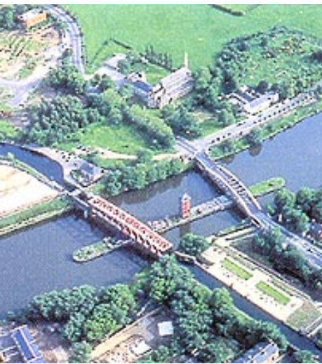
Aerial view of Barton swing bridge and the swing aqueduct, where the Bridgewater Canal crosses the Ship Canal.
